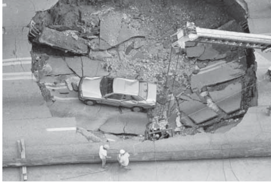
Figure 3 When land overlying a cavern collapses to form a sinkhole, human-made structures, such as this highway, can be damaged.
